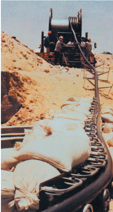
Installation of Power Cables
