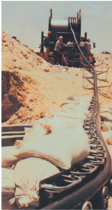
Installation of Power Cables
